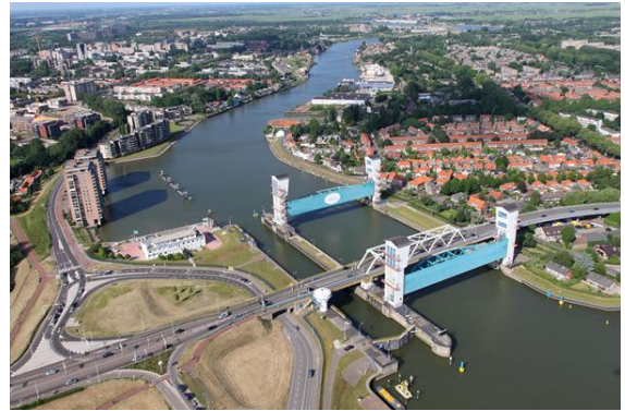
Figure 3: The Algra complex consisting of a lock, a bridge, and two storm surge barriers [https://beeldbank.rws.nl, Rijkswaterstaat / Joop van Houdt].
