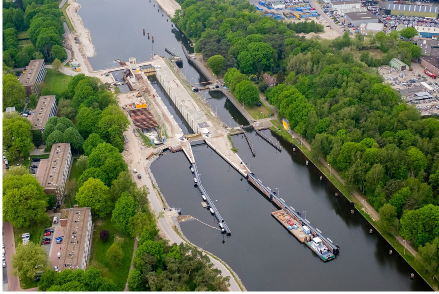
Fig. 3. Photo of Lock III, located at Tilburg, The Netherlands. Image from https://beeldbank.rws.nl , Rijkswaterstaat.
