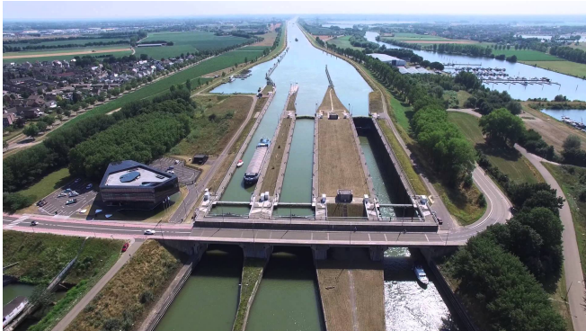
Fig. 2. Lock system in Maasbracht, the Netherlands.
