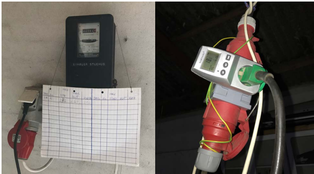
Figure 3. Examples of tinkering, additional power meter from H3 to keep track consumption (left) and homebuilt timer from H1 (right).
